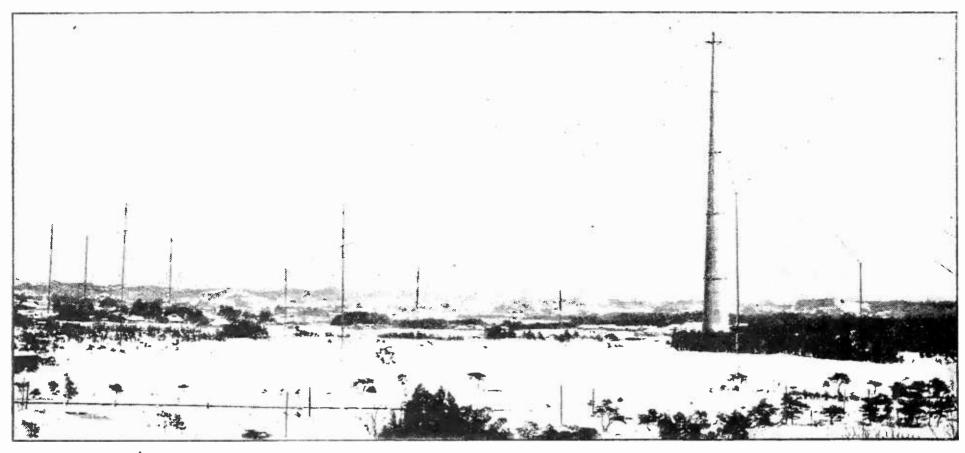
JAPAN'S ONLY IMMEDIATE MEANS OF COMMUNICATION WITH THE OUTSIDE WORLD This station, JAA, was erected in 1921. It is hard to appreciate from the photograph the size of the reinforced concrete mast. Its top is 660 feet above the ground, and the diameter of its base is sixty feet. A 500-kilowatt arc set is used, on a wavelength of 14,350 meters. Messages bearing news of the catastrophe and requests for aid were sent from this station via the land lines controlled at the receiving station at Tomioka
